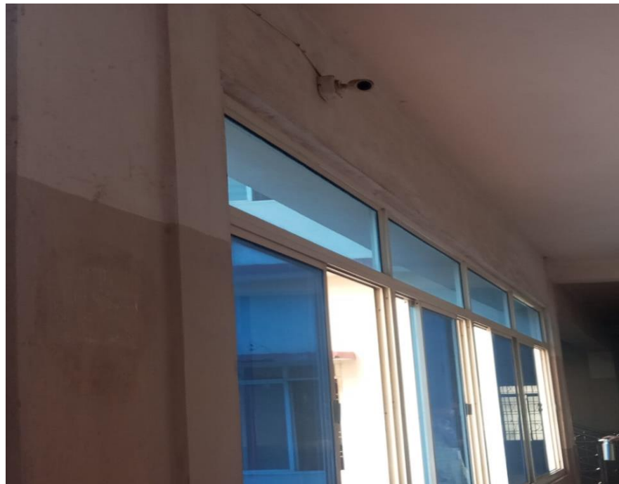
CCTV in Corridors
